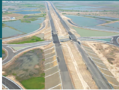
AHMEDABAD-DHOLERA EXPRESSWAY - DIAMOND CIRCLE
